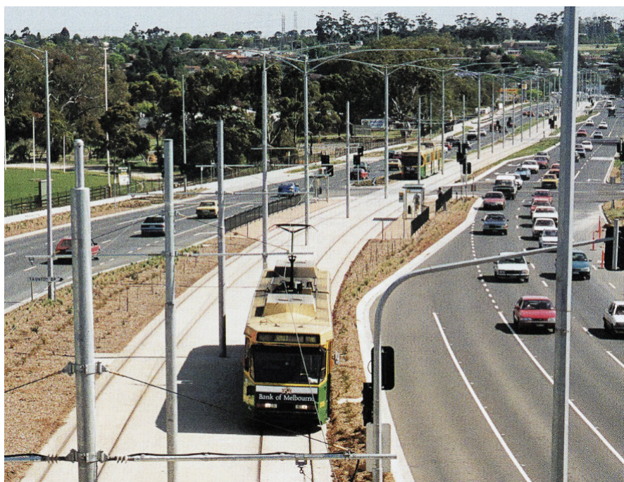
B2 class bound for the Bundoora RMIT terminus about to pass under the newly constructed Metropolitan Ring Road bridge, 1997. Photograph by Randall Wilson.
